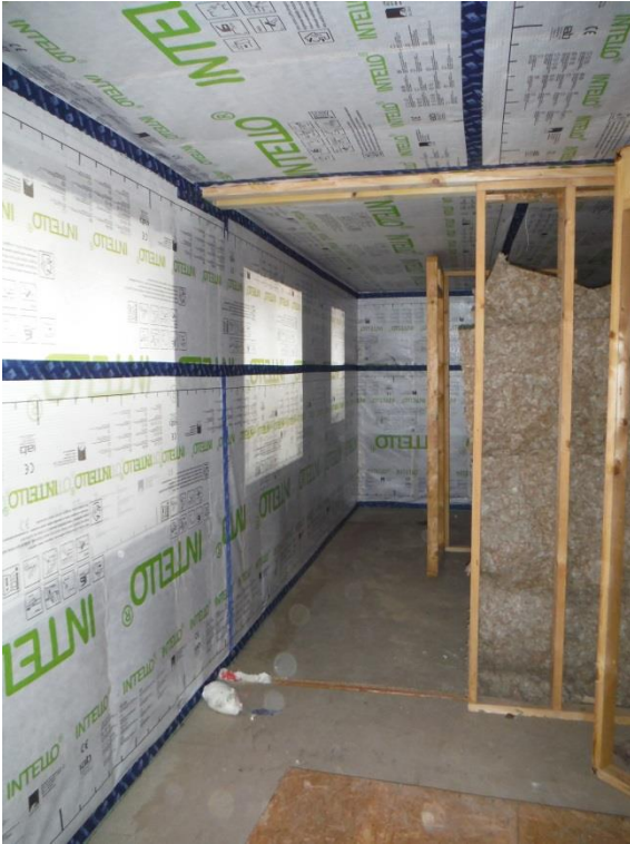
Figure 24: First floor, airtight membrane passes through party wall
