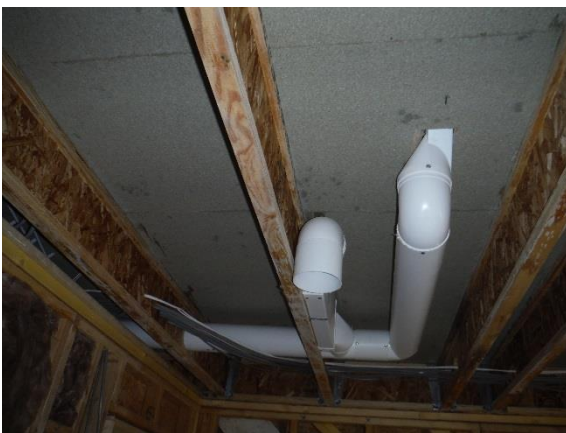
Figure 31: Ductwork in intermediate floor void
