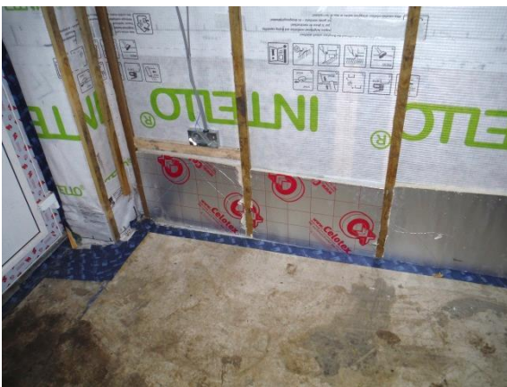
Figure 26: Membrane connected to airtight screed layer
