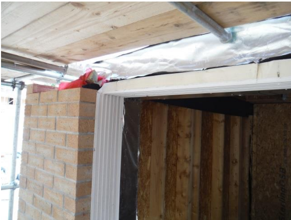
Figure 12: Door opening showing wall construction and insulated cavity closer
