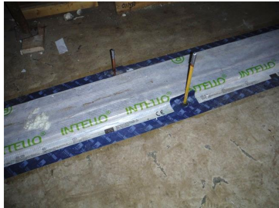
Figure 13: Party wall base; aerated blockwork plinth spanned by air membrane
