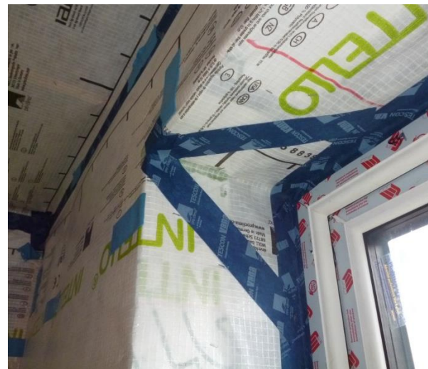
Figure 23: Window/wall air barrier junction
