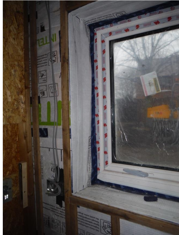
Figure 25: Airtight tape connects window frame to membrane
