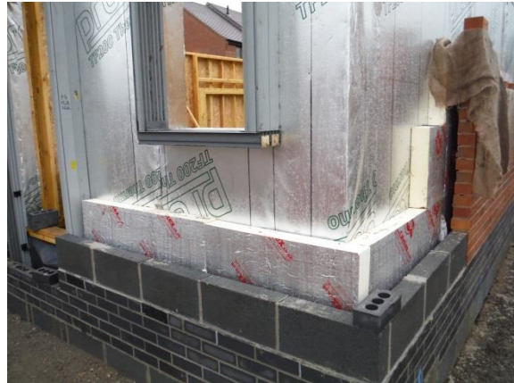
Figure 11: Construction of wall corner: brick finish to the right and the blockwork to be rendered
