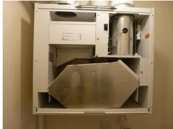
Figure 30: MVHR unit with cover removed
