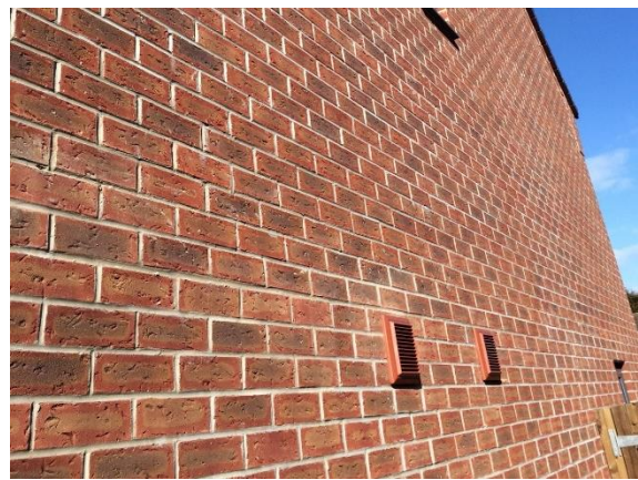
Figure 32: Intake and exhaust terminals
