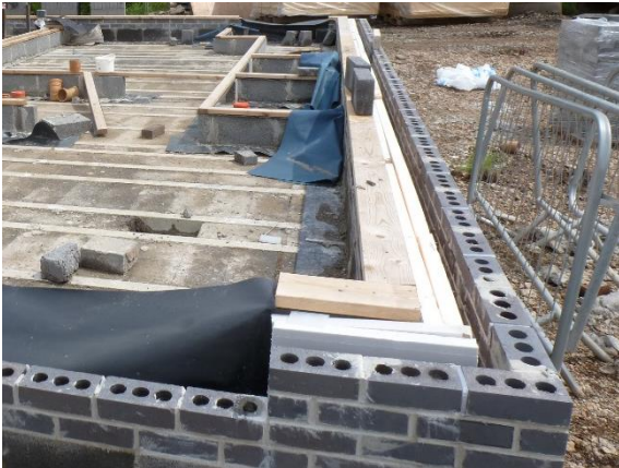
Figure 10: Suspended concrete floor, and wall built to plinth block height
