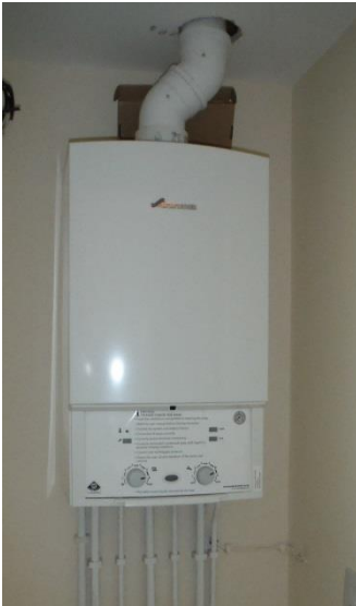
Figure 36: Boiler in upstairs store room
